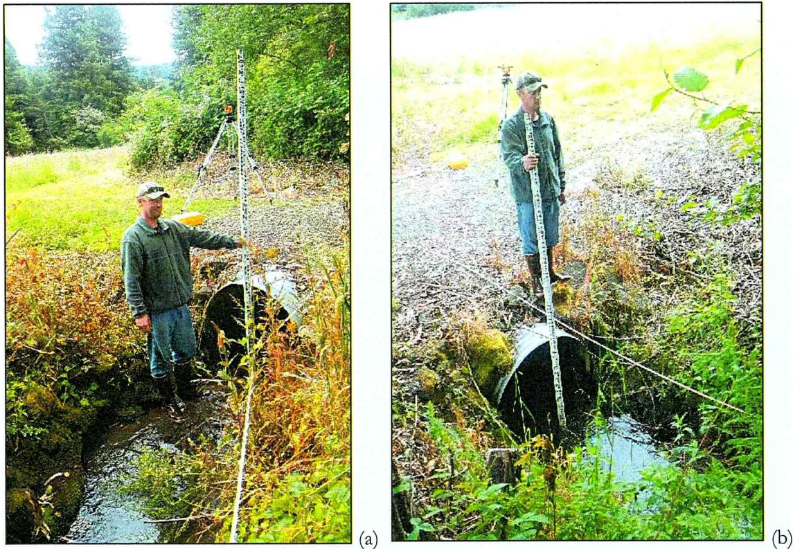
Figure 3-2: Existing CMP stream crossing set at a reverse grade with RSP along both banks, (a) outlet slightly embedded and poorly aligned, and (b) poor inlet alignment and aggradation upstream of culvert. Photo courtesy of SRA.
