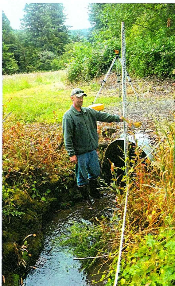
Crossing #2: Existing CMP stream crossing set at a reverse grade with RSP along both banks, outlet slightly embedded and poorly aligned, and poor inlet alignment and aggradation upstream of culvert.
