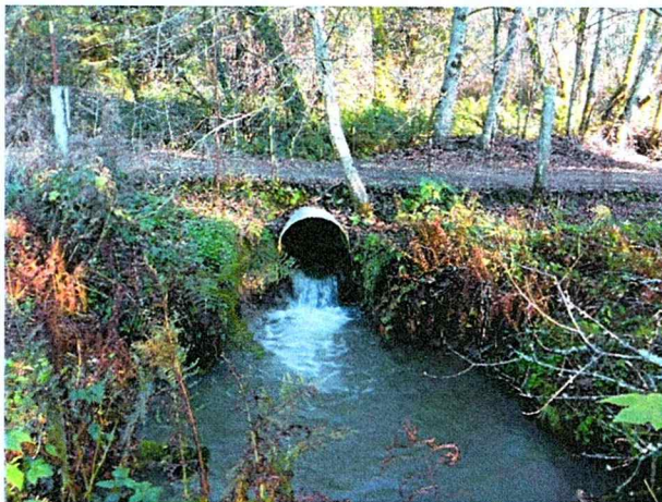
Crossing #1: Existing CMP at crossing #1 with a water surface drop at outlet during low winter flows and poor inlet alignment and aggradation upstream of culvert.
