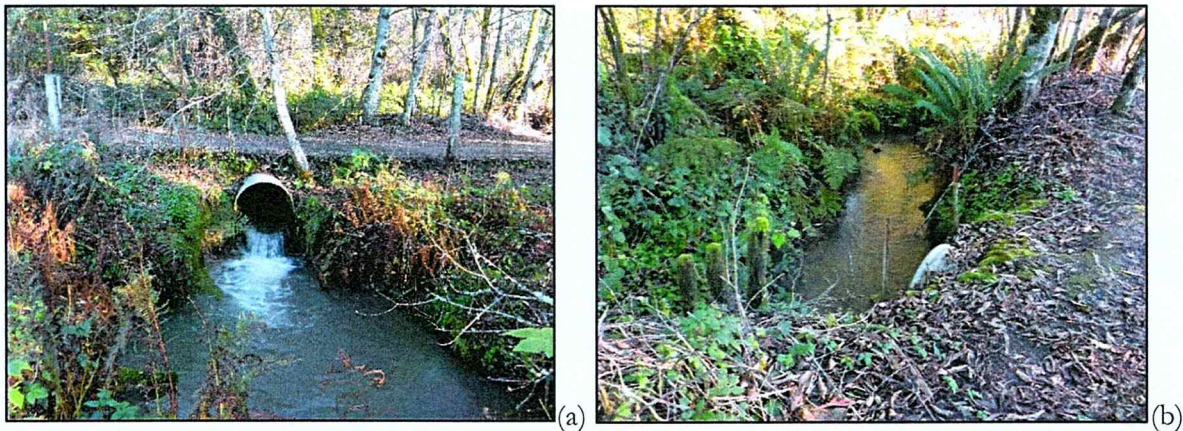
Figure 2: Existing CMP stream crossing with (a) water surface drop at outlet during low winter flows and (b) poor inlet alignment and aggradation upstream of culvert.
