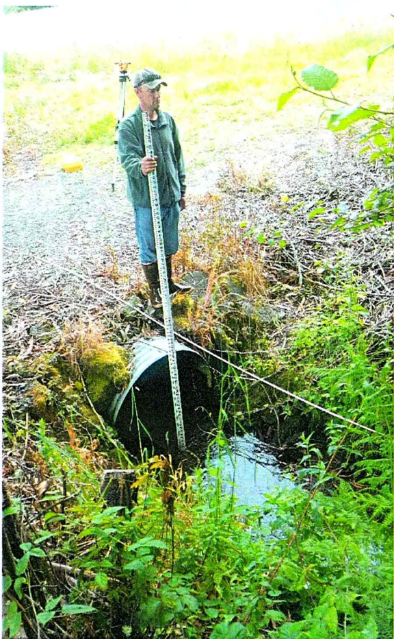
Crossing #2: Existing CMP stream crossing set at a reverse grade with RSP along both banks, outlet slightly embedded and poorly aligned, and poor inlet alignment and aggradation upstream of culvert.
