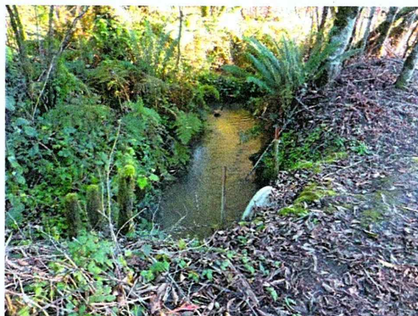
Crossing #1: Existing CMP at crossing #1 with a water surface drop at outlet during low winter flows and poor inlet alignment and aggradation upstream of culvert.
